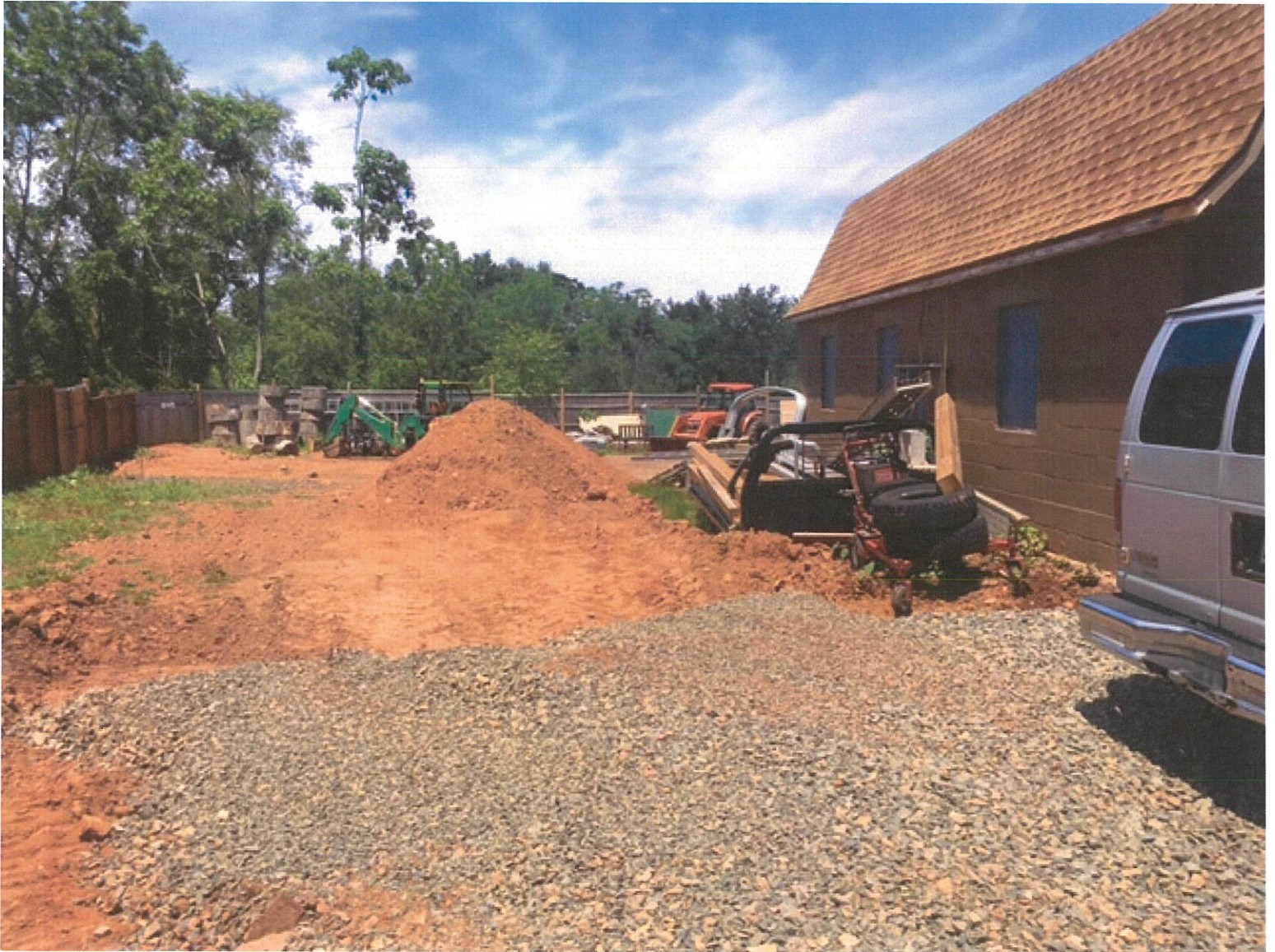
Blight Photos 1 Bassett Road 06/10/2021
